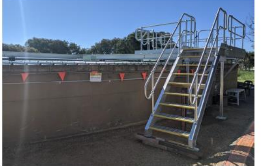
TK-01 – Para Vista Tank Safe Access installation
