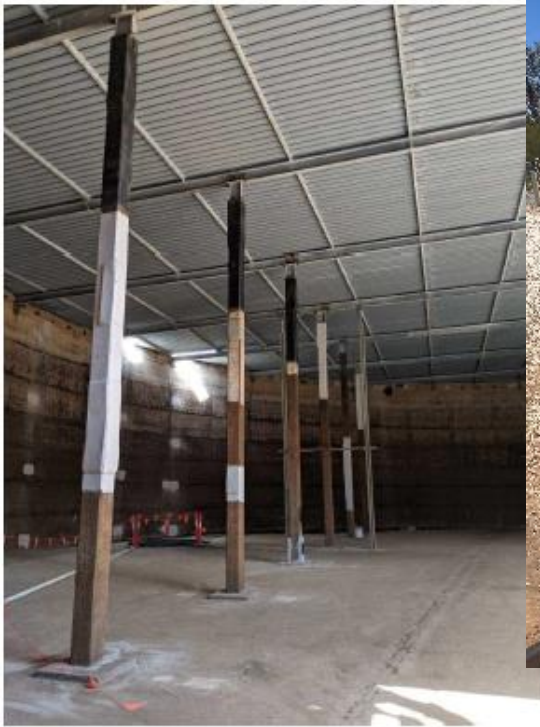
TK-01 – Para Vista Tank Internal Concrete Column Remediation
